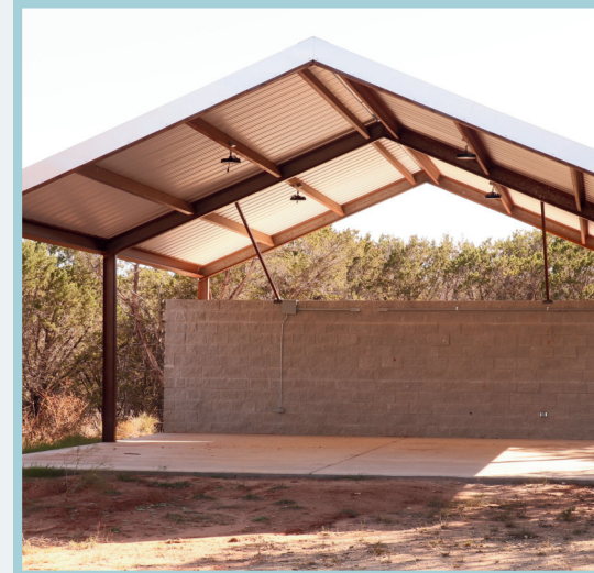
Newly Built Pavilion with Restrooms
