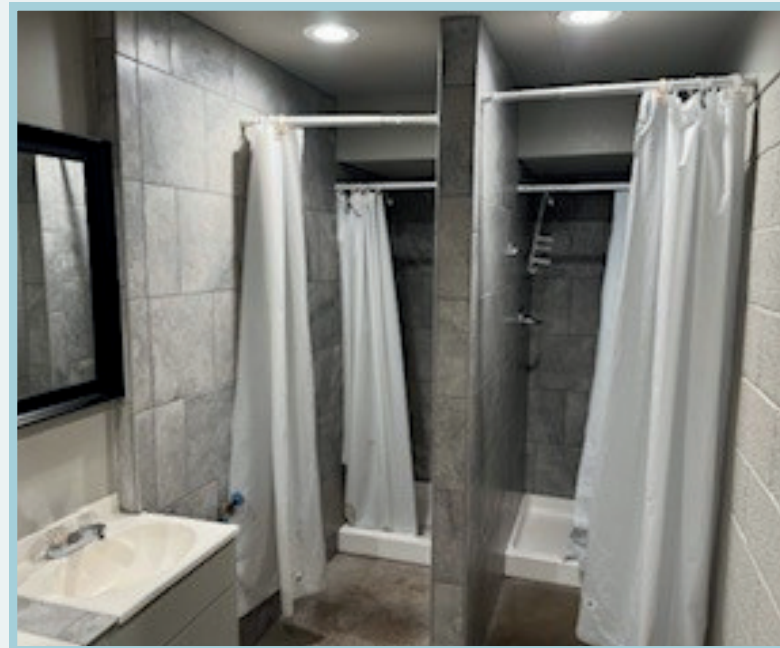
Shower Stalls After Renovation
